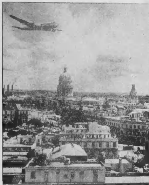
Shown above is the Cuban capitol building in Havana. The dome of the famous structure was modeled after the United States capitol in Washington, D. C.
